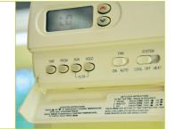
Setting your thermostat to the "On Position allows your fan to circulate air continuously when not in a heating or cooling mode.
